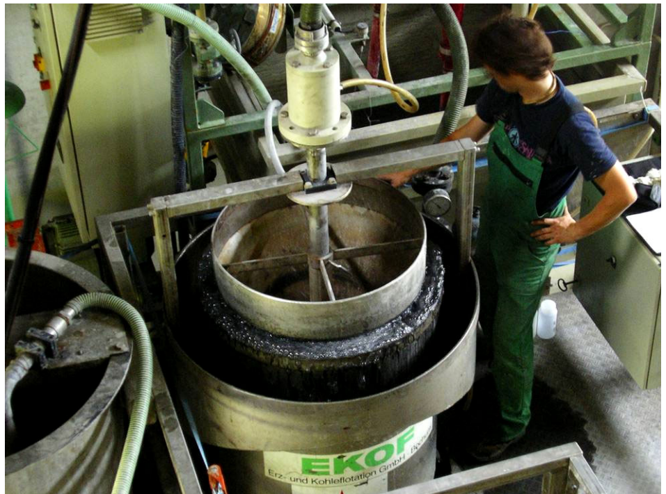
Fig. 1: operation of a flotation pilot plant at KEBAG, Zuchwil
